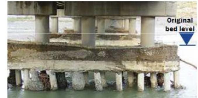
**Contraction scour:** the result of water accelerating as it flows through an opening (bridge) that is narrower than the channel itself
