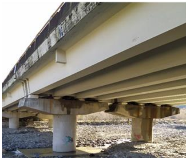
Figure 11. Bridge B: general view.
